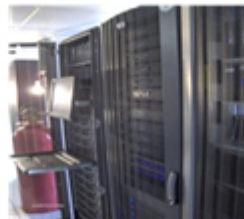
Rack assembly and hardware installation
